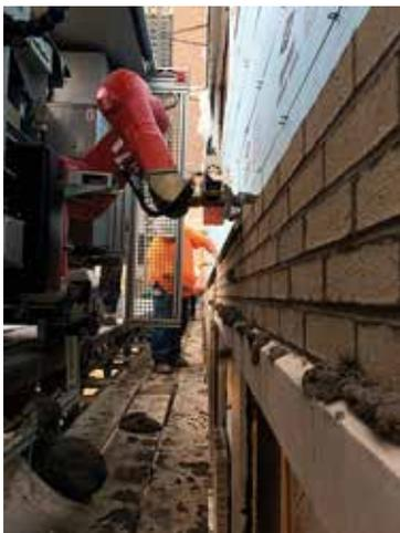
Fig 3 Construction Robotics, SAM 100
