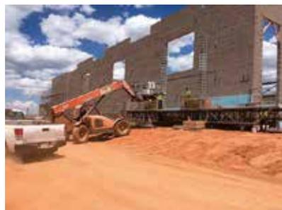
Fig 4 Construction Robotics, SAM 100, Laramie
