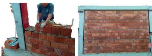
**Fig 5** Posa in opera e vista finale del sistema a giunto in gomma deformabile (Padova, Italia) / Installation and final wall of the deformable rubber joint system (Padova, Italy)
