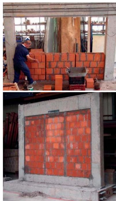
**Fig 6** Posa in opera e vista finale del sistema a giunti verticali (Grecia) / Installation and final wall of the vertical joints system (Greece)
